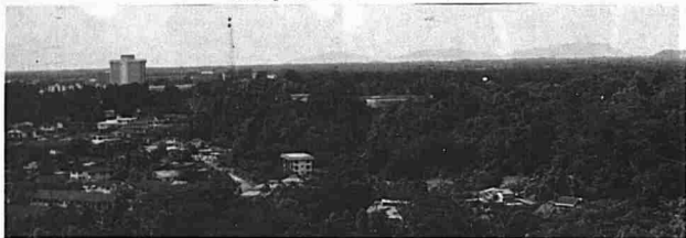
The steel reservoir on Bukit Tuan Muda along the Bampfylde Road
