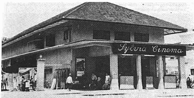
The original look of the Sylvia Cinema before it was demolished to give away to the Third Secretarial Office building.
