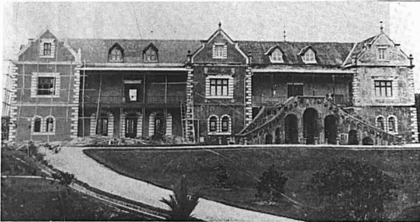
The new wing of the museum was constructed in 1911. The large flight of the brick work steps outside the centre of the old wing was removed by order of the Rajah in 1912.
